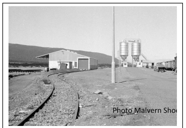
Cement silos & good shed for the Tongariro Power Scheme
